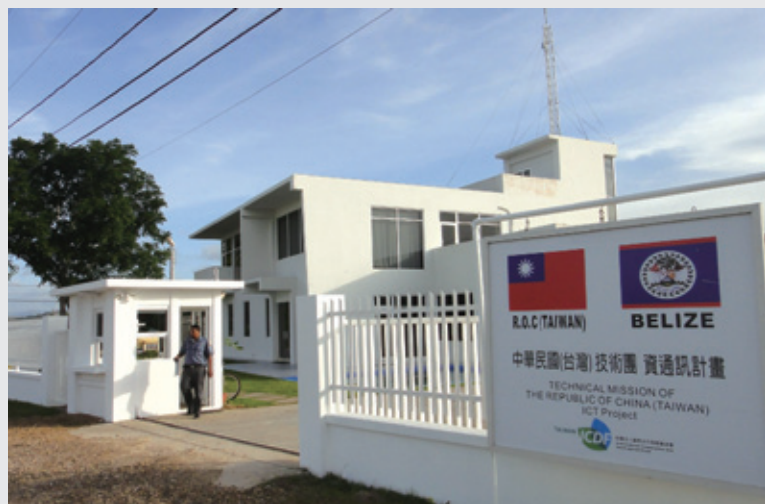
▲ The National ICT Center in Belize, built with assistance from the TaiwanCDF. The development of e-government systems and the provision of ICT training at the center have made the site a hub for the promotion of ICT development.
